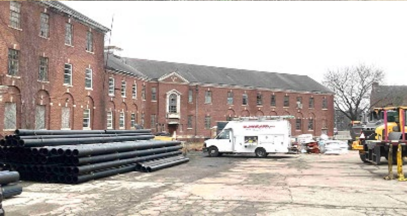
Water Main Replacement, Fairfield Hills Campus - Newtown, CT
