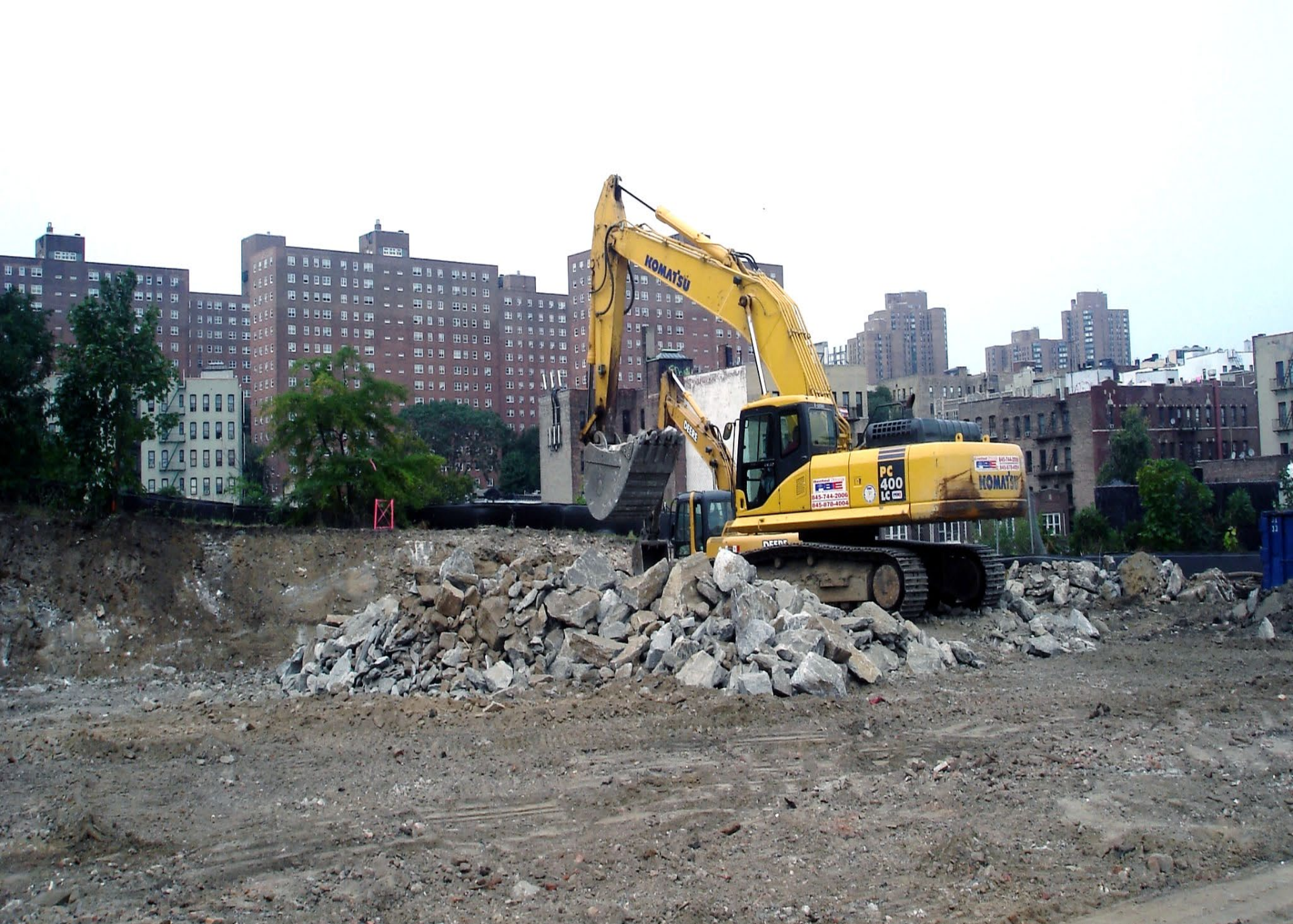
West Bronx Tank Removal – Bronx, NY
