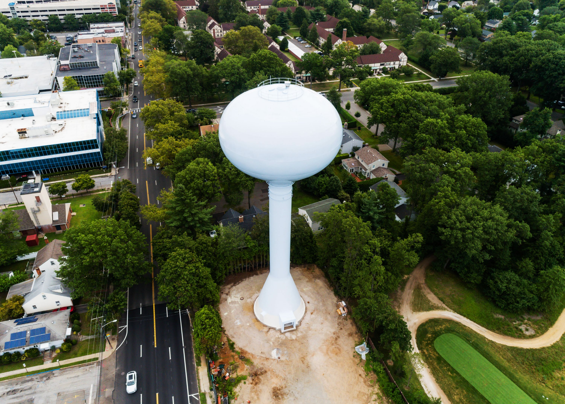
Incorporated Village of Garden City Road Tank Replacement – Garden City, NY
